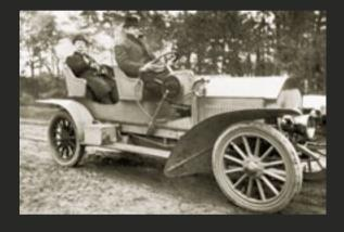
Alternative drive systems are not a thing seen only in the 21st century. In 1908 the founder of the Czech electrical engineering industry and famous inventor František Křižík bought an L&K, type E, to fit it with a hybrid system (petrol and electricity). In the picture, the power control is under the steering wheel, on the driver's right-hand side.
